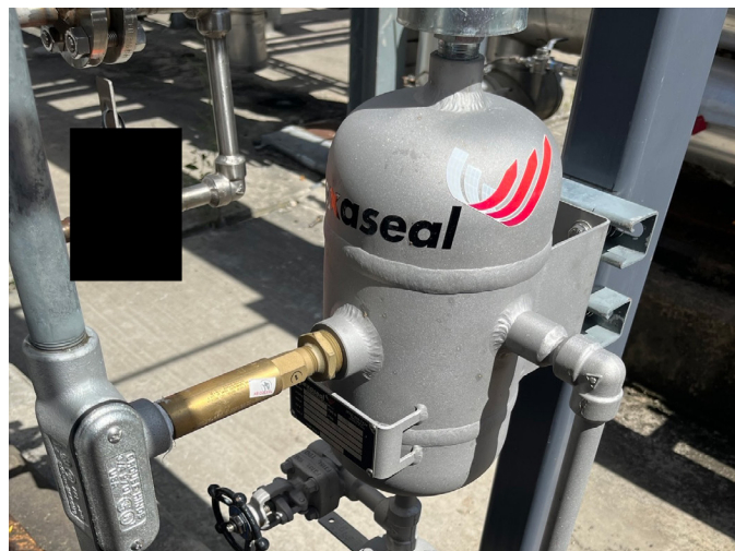
Figure 5. API Plan 65A reservoir
